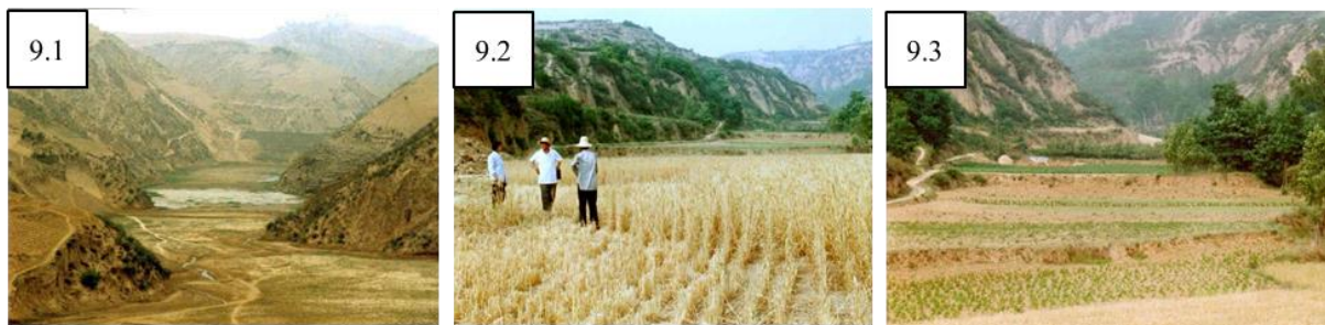
Picture 9. The lower check dam is an earthen wall some 2 meters high; it is collecting the silt released from the higher flood mitigation dam. 9.1). At Shanxi, Mizhi, Yulingou gully (China) 9.2 and 9.3). Fenxi county, Shanxi (China) Source: Planting Water, 2012
