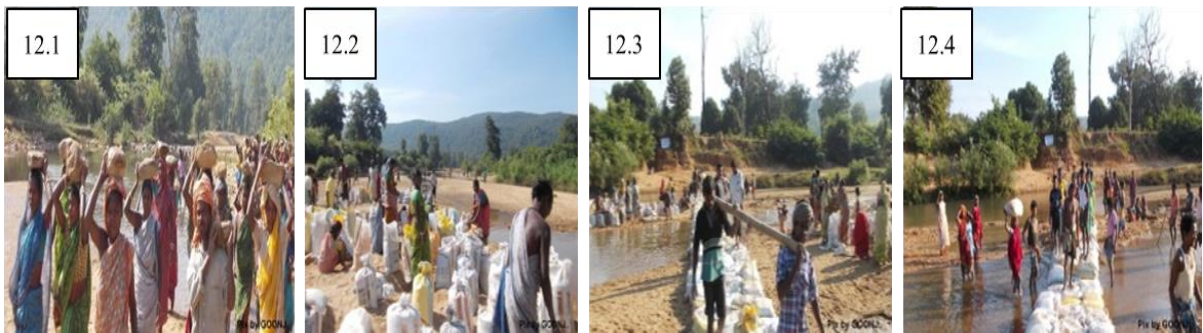
Picture 12. The peoples of India were making local check dam at the same time of bridge by sand bag structure at Telkoi Block of Keonjhar, Odisha Source: Goonj, 2012
