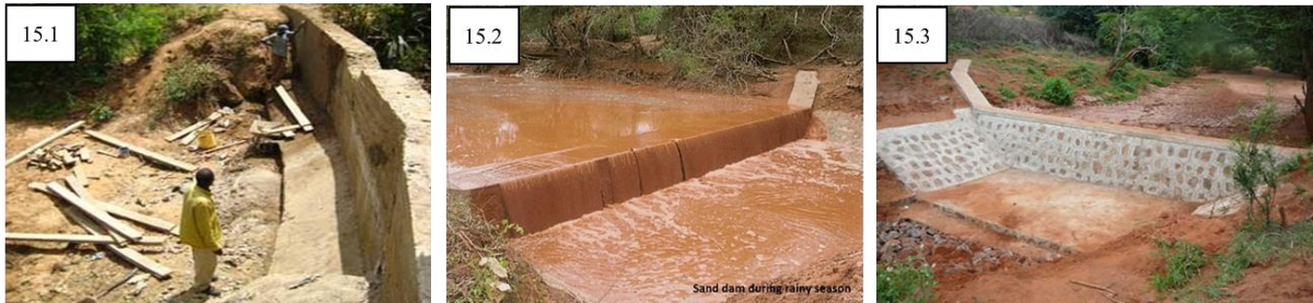
Picture 15. The sample of smallest dams or sand dams in Kenya
