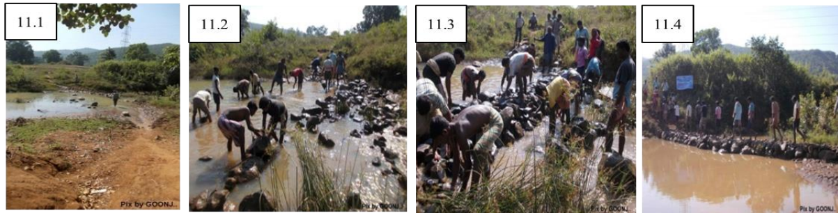
Picture 11. The peoples of India were making local check dam at the same time of bridge by rock structure at Bhaliadihi village, Keonjhar, Odisha Source: Goonj, 2012
