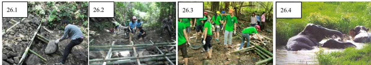
Picture 26. Check dam making aiming to slow down the stream and trap the sediment. The main structure of the check dams made by bamboo as a cage with 50 cm. high, a crossing the stream at every 5 - 10 meter apart from each other. Providing drinking water and bathing areas for wild elephants.
