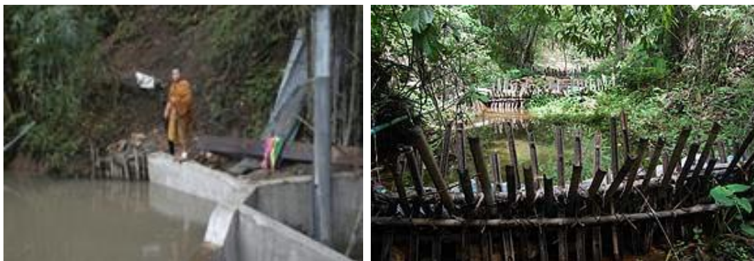
Picture 28. The sample of various local check dam which initiate by monk.
