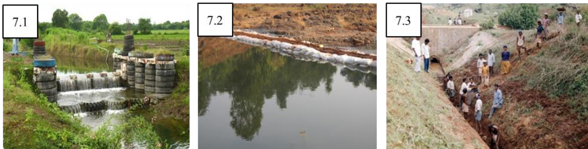
Picture 7. The sample check dams or temporary dam in India as 7.1).The check dams were constructed from vehicle tires, sand, stones, cement, bamboos and plastic micro concrete. 7.2).Vanrai Dam 7.3).Tabelagummi Dam
