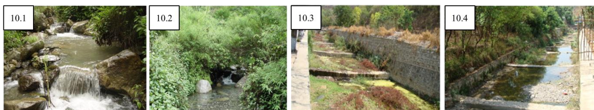
Picture 10. The sample of rock dams and concrete check dams in southwestern China. (Shengou Creek, Jiangjia Ravine and Xiaobaini Ravine) Source: Yu, et.al., 2012
