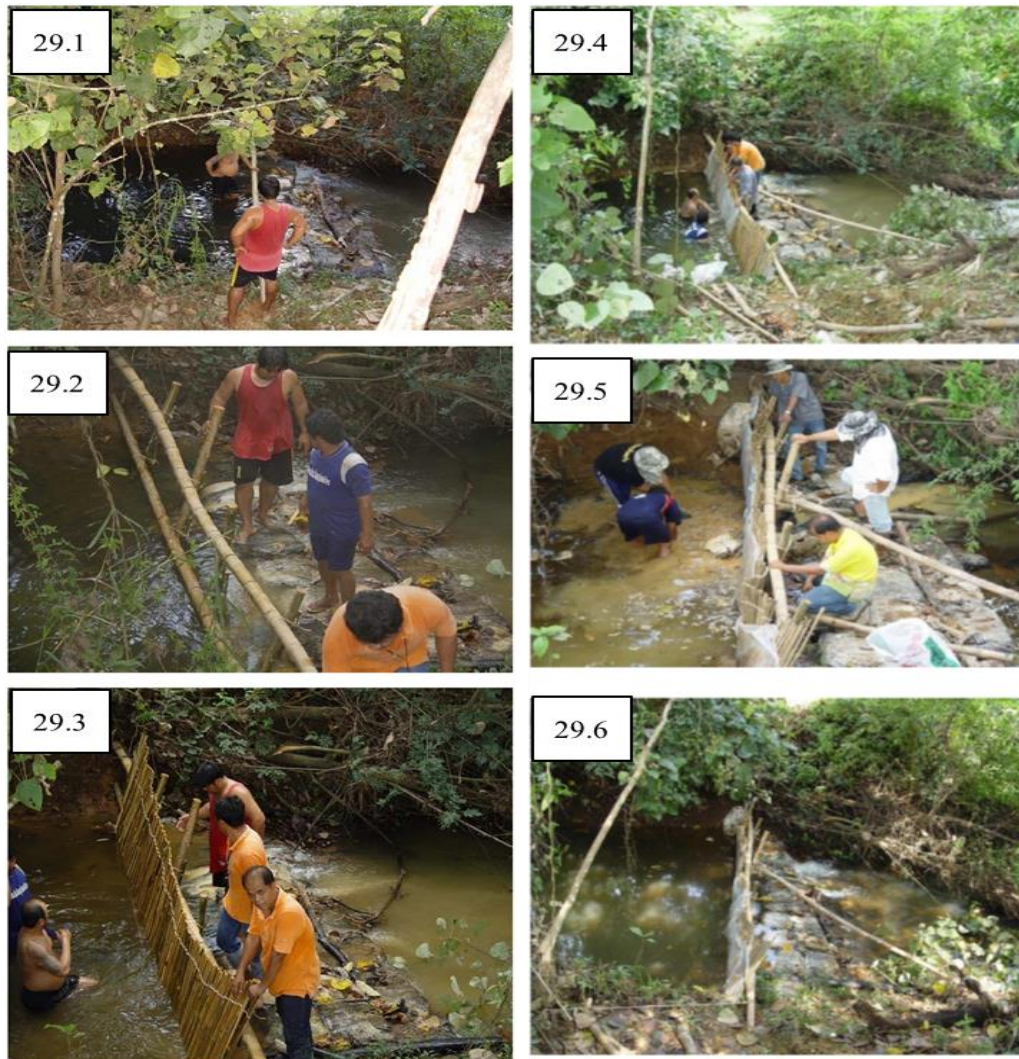
Picture 29. Step of making low cost check dam material utilization following
