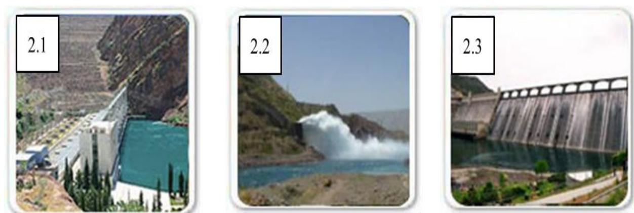
Picture 2. The sample of Top Three highest dam in the worlds as 2.1).Rogun Dam (Tajikstan) 2.2).Nurek Dam (Tajikistan) 2.3).Grand Dixence (Switzerland) Source: A Short Encyclopedia, 2010.
