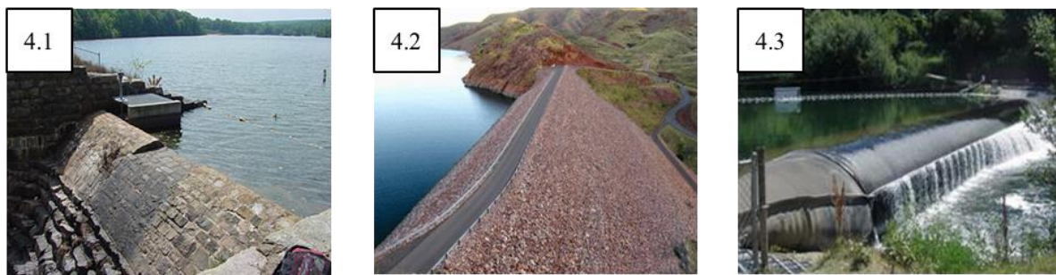
Picture 4. The sample of semi-permanently dam make from 4.1). Rock 4.2). Earth and 4.3). Rubber Source: Small Dam Gallery, 2011, Newton Consultants, Inc., 2011 and U.S. Geological Survey, 2011.
